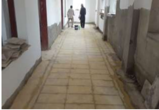
Tiling of Ground and 1 st floor
