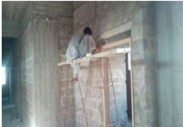
Door Frames of Ground Floor Being Fixed
