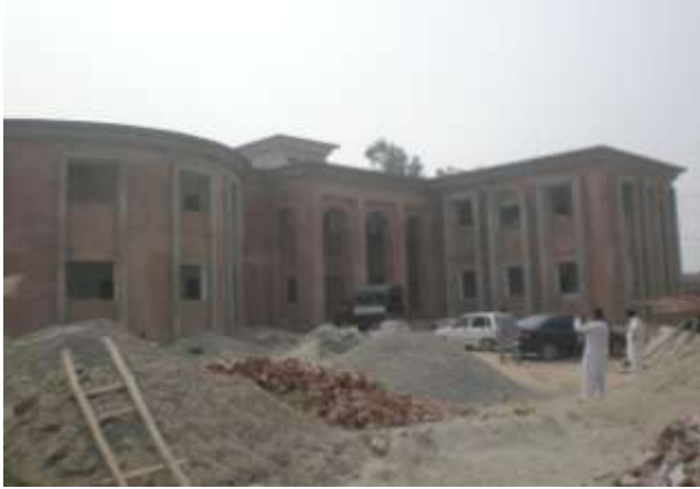
MATRC Peshawar - Grey Structure Completed
