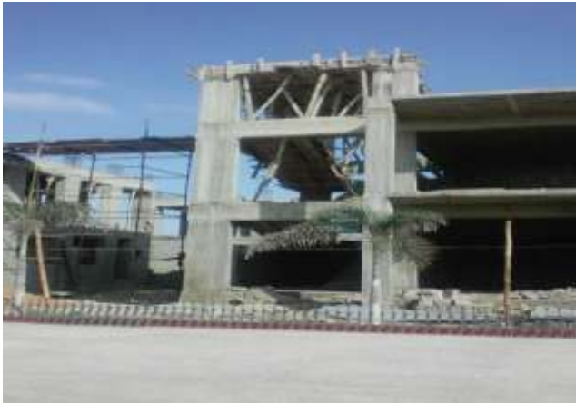
Shuttering of 1st Floor Removed
